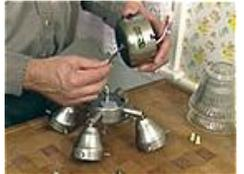
6. **Secure.** Finally, lift the light fixture into place, and secure it to the motor assembly. Turn the power back on, and cool off.
