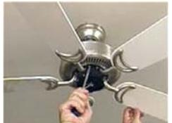
5. **Install light fixture** to the switch housing. The manufacturer of the fan will provide specific instructions for the electrical wiring.
