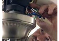
4. **Raise the canopy** up to the ceiling to cover the receiver and wires and fasten it with screws. Assemble the blades and blade carriers. The blades simply attach to their brackets with screws. Mount the blades to the bottom of the motor
